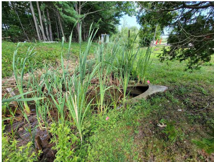
Photo 1. Culvert entry looking east toward access road
