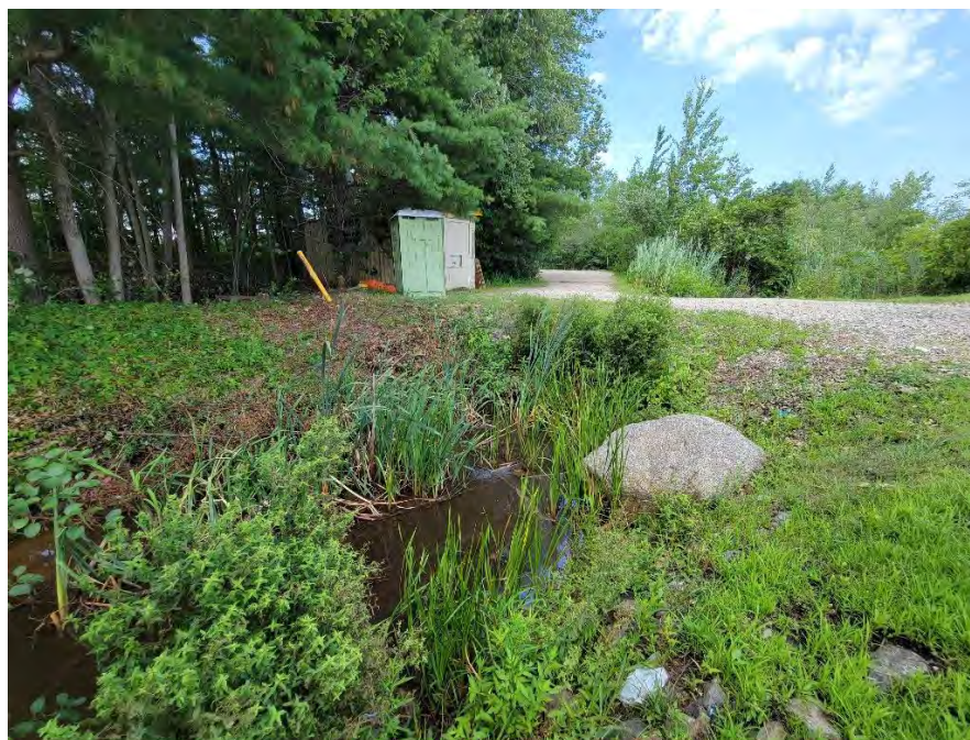
Photo 2. Culvert entry from the west of access road
